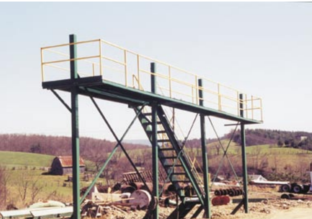
Fig. 1: Tarping station at a Virginia sawmill.
