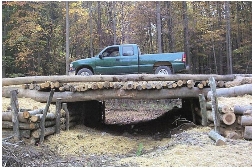
Fig. 1: Log bridge side view.
