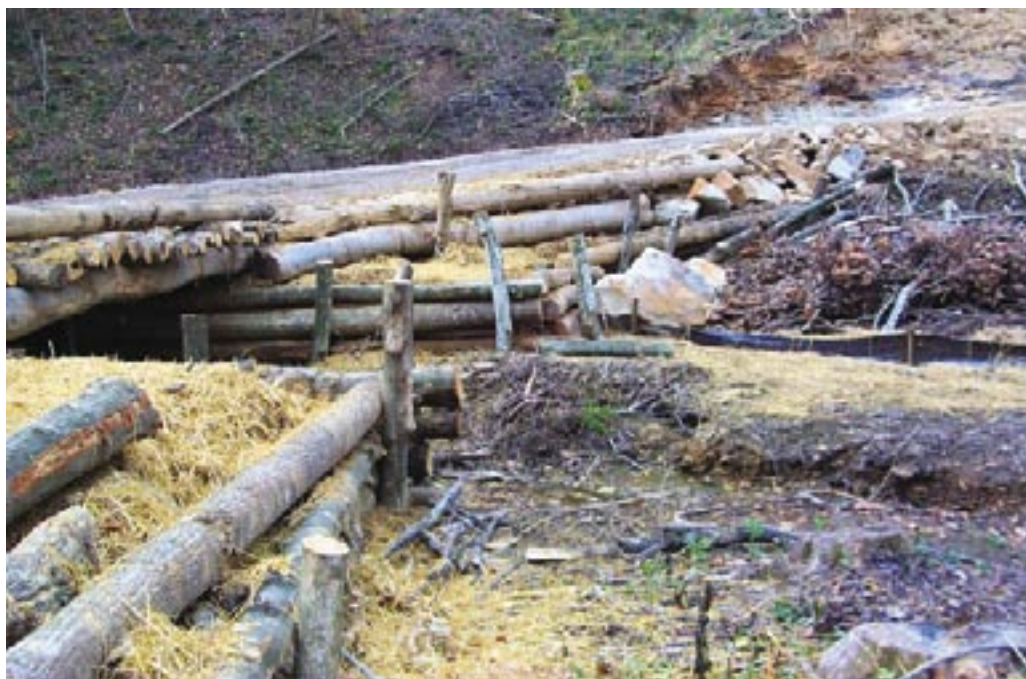
Fig. 2: Log bridge abutments.
