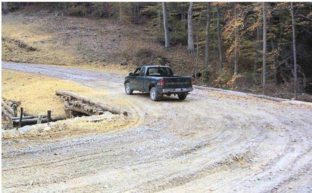
Fig. 3: Log bridge provides cost-effective access.
